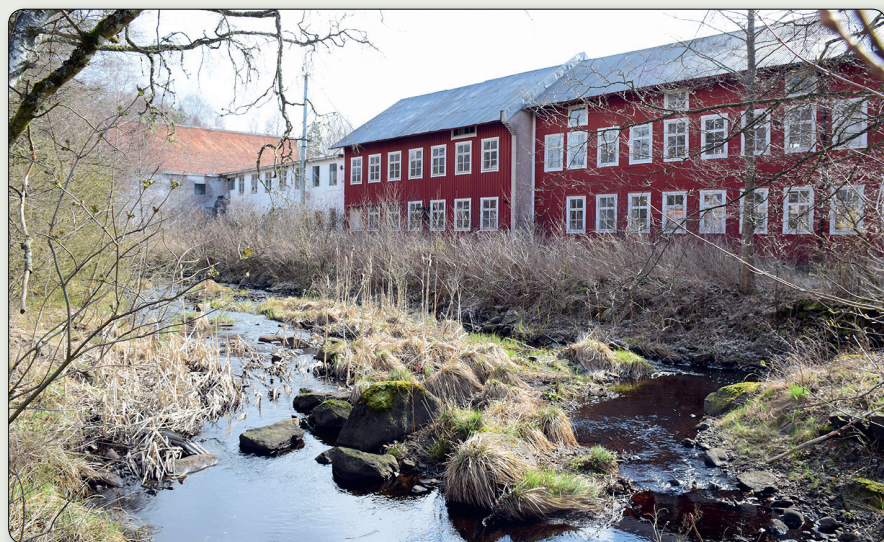
The old chair factory is located close to the river Linneån. Photo: Jönköping County Museum.
