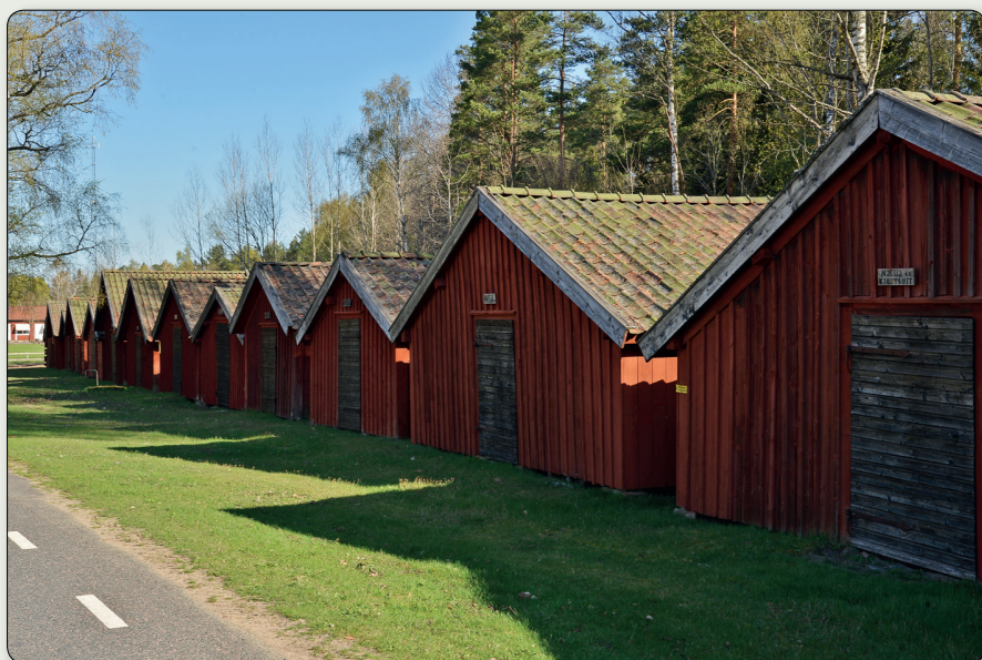
Åker Church Stables. Photo: Jönköping County Museum.
