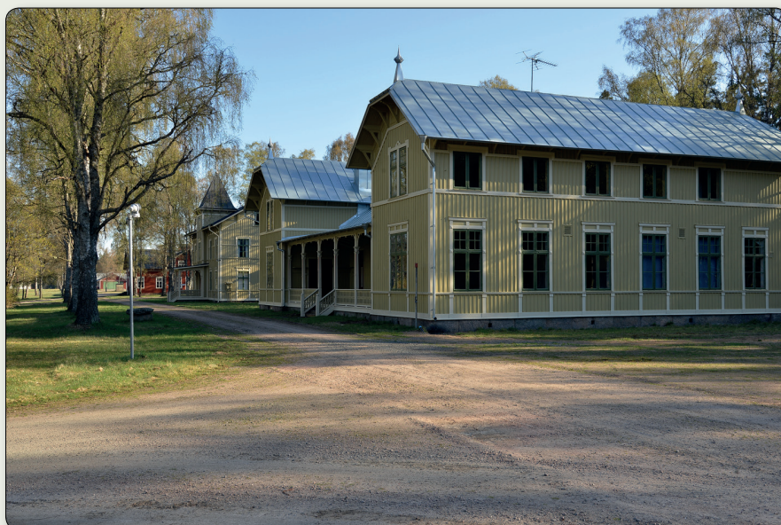
The buildings in the Western Camp are mainly from the period late 1800 to early 1900. Photo: Jönköping County Museum.
